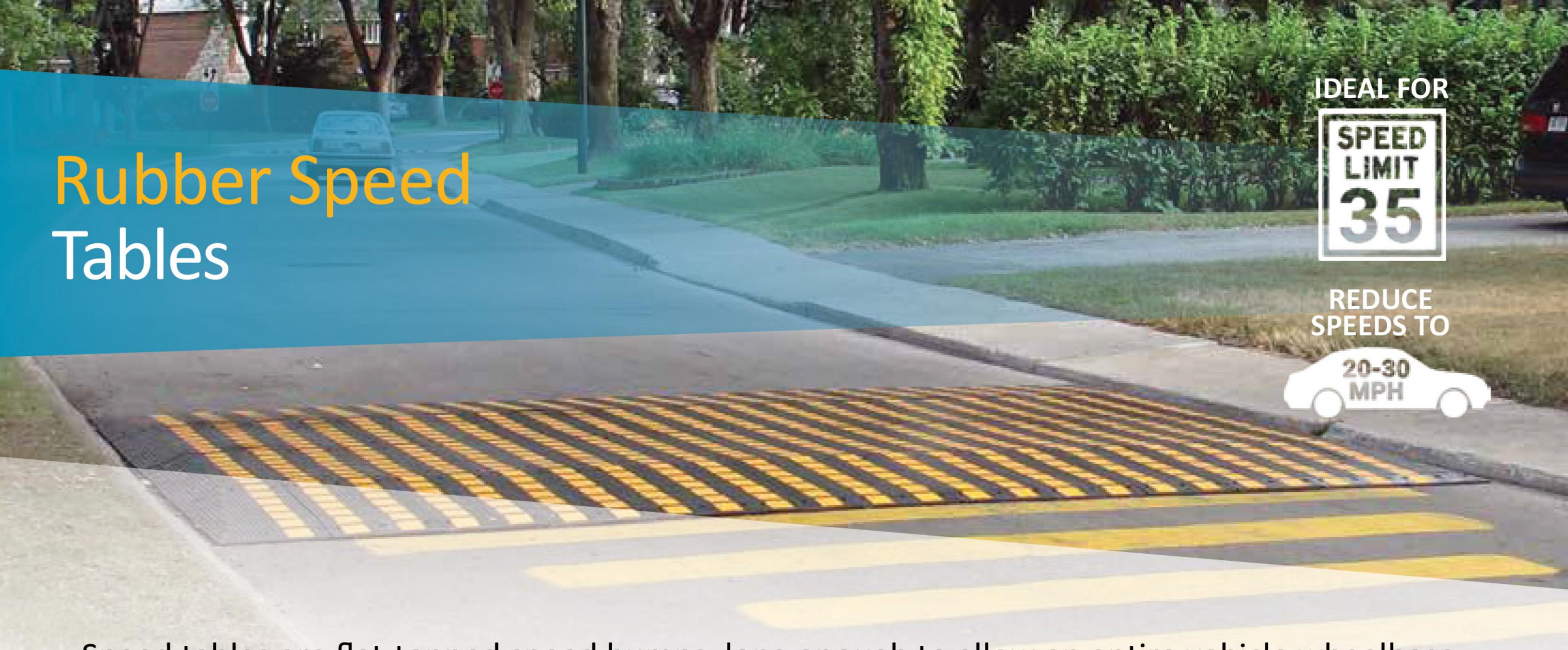
Speed tables are flat-topped speed humps, long enough to allow an entire vehicle wheelbase to rest on top of the table. The flat top design slows vehicles more gradually than speed humps, allowing traffic to pass at speeds of 20-30 mph. Speed tables are an ideal solution for residential roads where the goal is to maintain traffic flow while reducing speeding.
