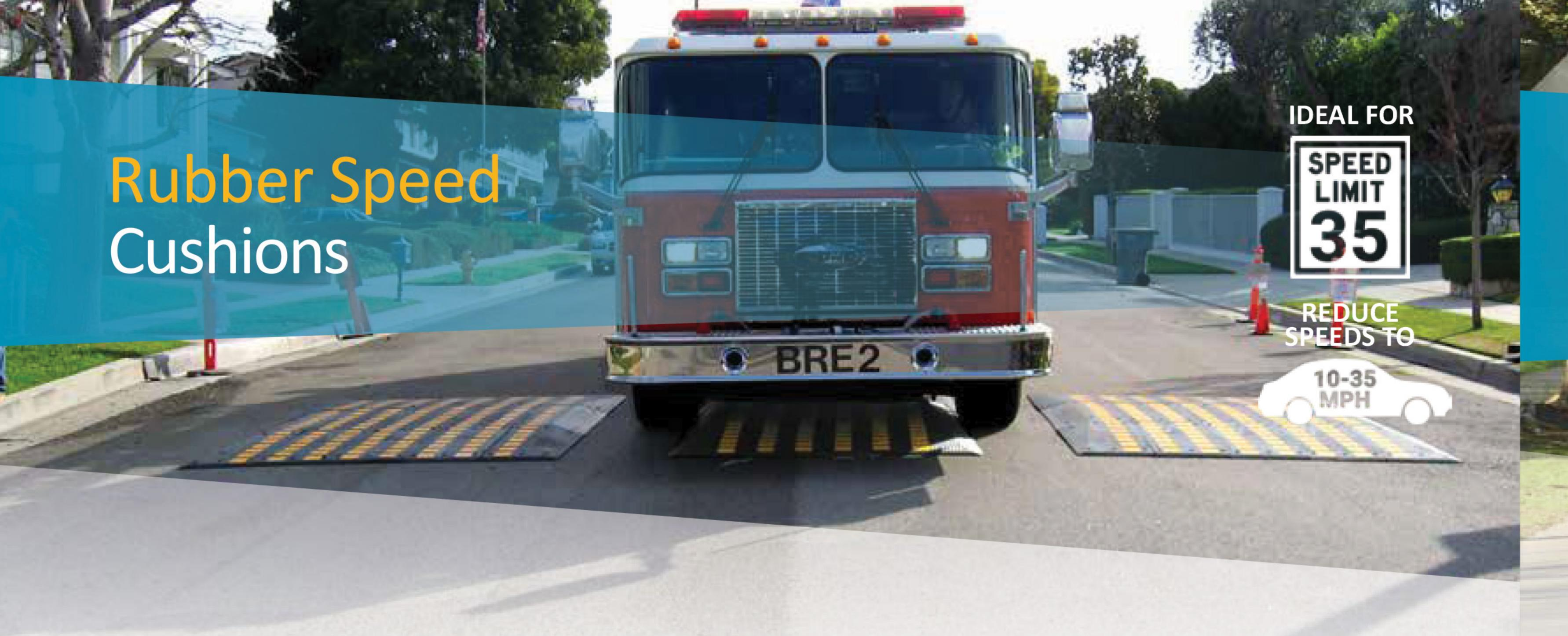
Speed cushions are raised devices similar to speed humps but with narrower widths. They are designed to slow cars without affecting emergency response time. The wider wheel base of emergency vehicles allows them to straddle the cushions while other vehicles must ride over them, slowing down to pass. Speed cushions are placed across the width of the road.
